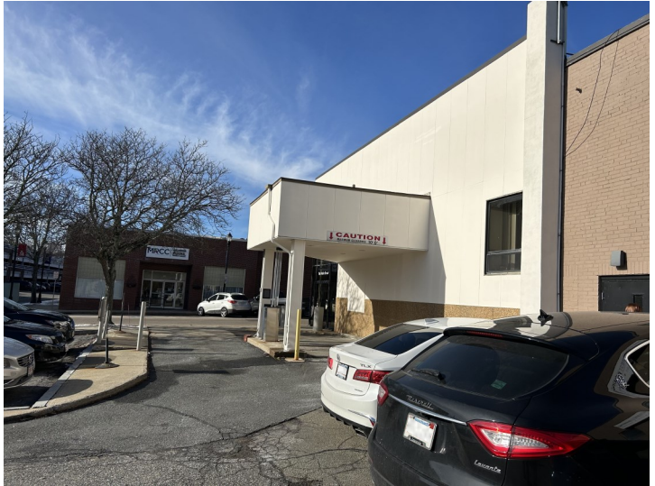
Former Bank Drive-thru
